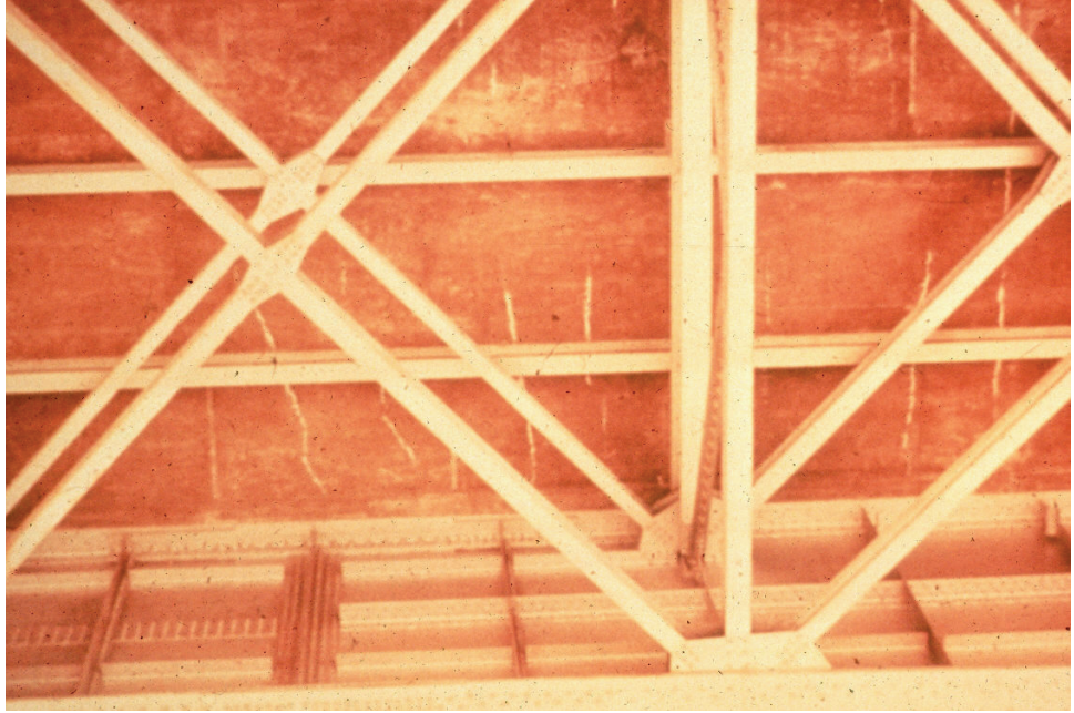
Figure 2.2.13 Transverse Cracks
