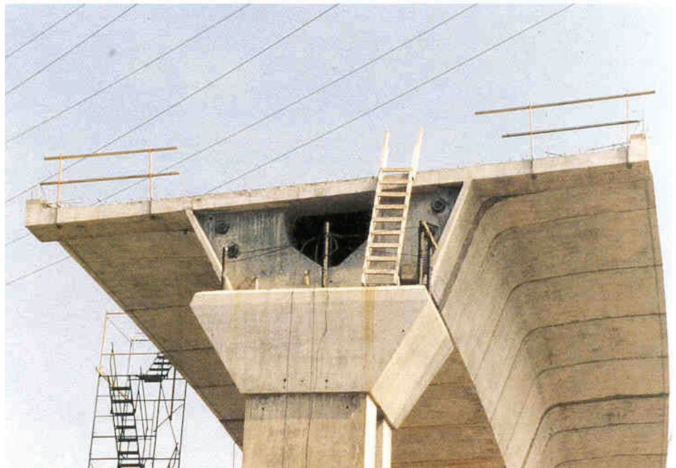
Figure 2.2.5 Post-tensioned Concrete Box Girder
