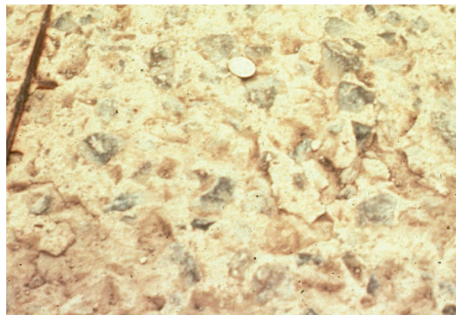
Figure 2.2.19 Severe Scaling
