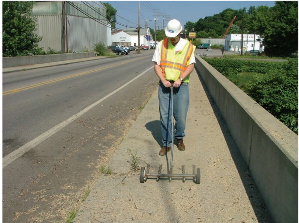
Figure 2.2.29: Inspector Using a Chain Drag
