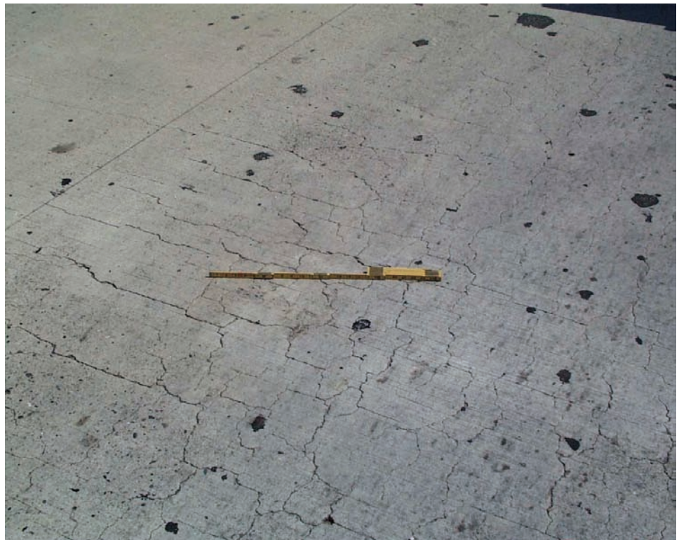
Figure 2.2.12 Shrinkage Cracks
